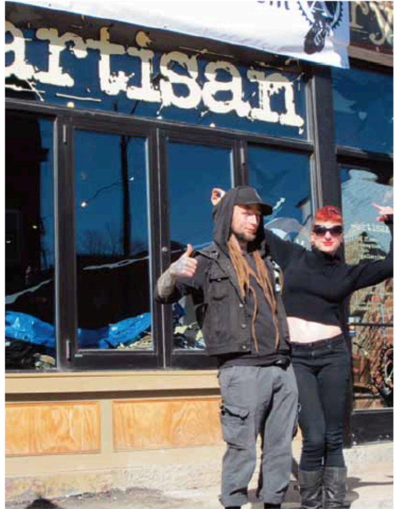
ABOVE: Jason and Mel Angst, owners and operators of Artisan Tattoo (5001 Penn Ave.) in Garfield, try directing foot-traffic into their store while also completing a massive building renovation project. Photo by Andrew McKeon.
